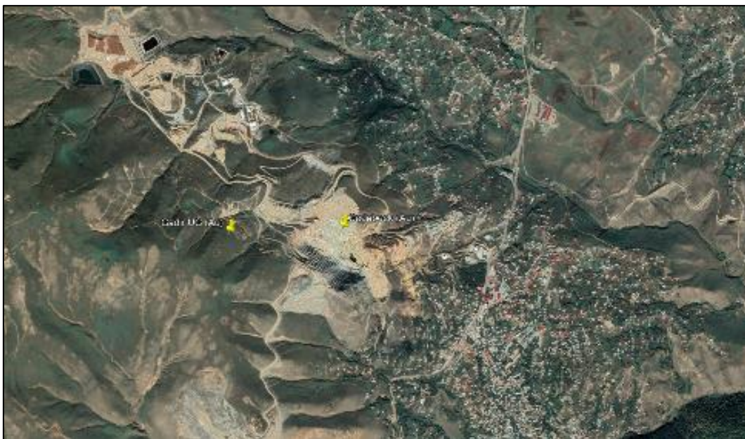
Figure 9: Gedabek open pit (centre) with location of Gadir UG mine illustrated. Heap leach, AGL and FLT facilities located to NW and Gedabek city to the SE.
