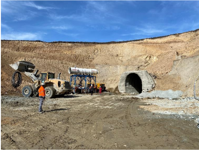
Box cut and portal at the Gilar underground development
